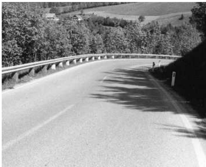
On a French road, a second lower flat rail is fitted under the armco (above: rail seen from behind)
